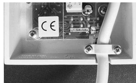
Carefully fit the control plate into the back box ensuring that no wires are trapped during the siting process.
